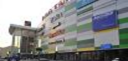
Galleria Arad, Arad, Romania
