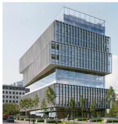
Advance Business Center Sofia, Bulgaria
