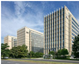
Korona Office Complex, Krakow
